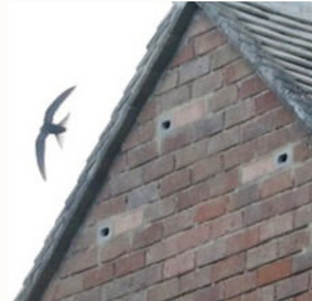
'Universal bricks' integrated within the building's fabric.
